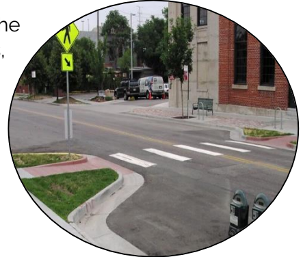
Curb extension example. Image Credit: Richard Drdul
